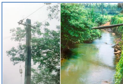
Figure 1: The overhead electric line from which the electricity was diverted is seen on the left. The nearby stream where the deceased was electrocuted is seen on the right. The wire was dropped down near the coconut tree trunk and the deceased was standing downstream.
